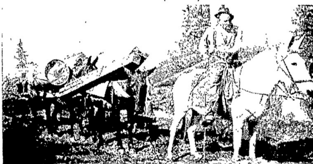
A packer hauling in timber for the tower.
