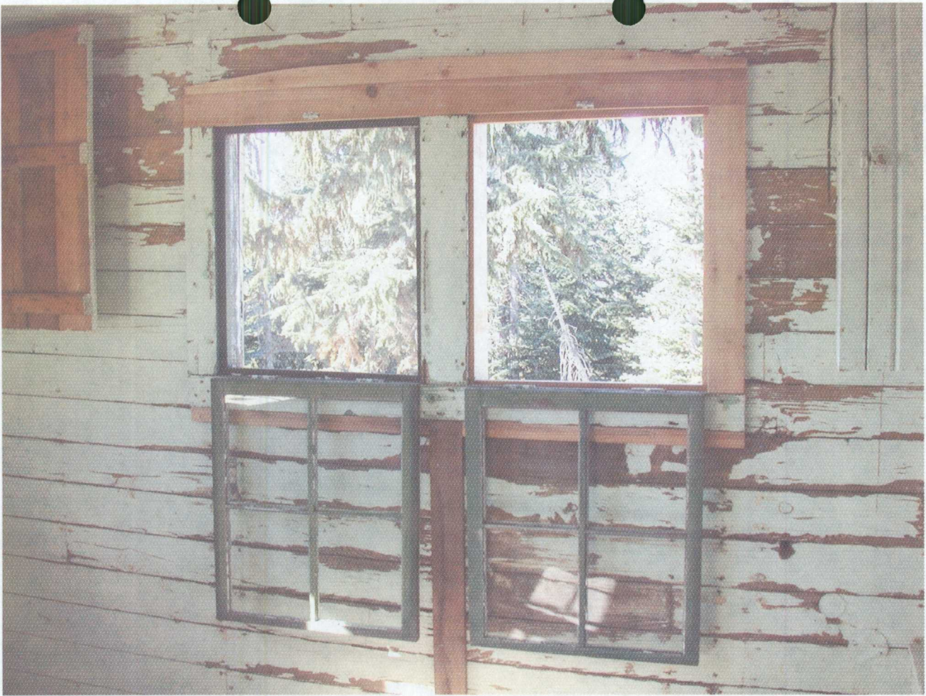
Trim repairs and scraped west wall
