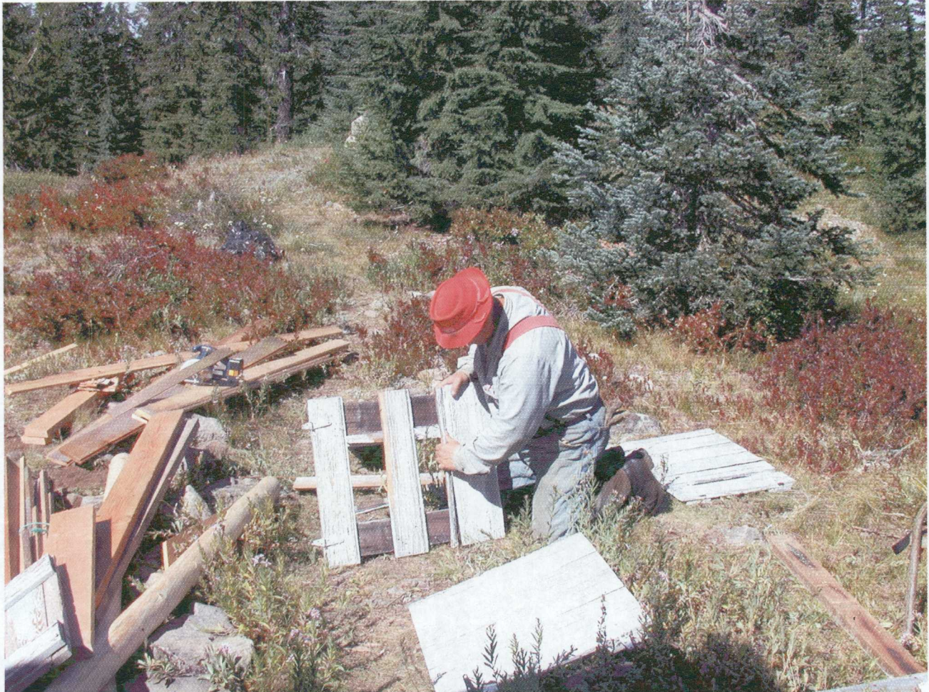
Gary McCullough repairing storm shutters
