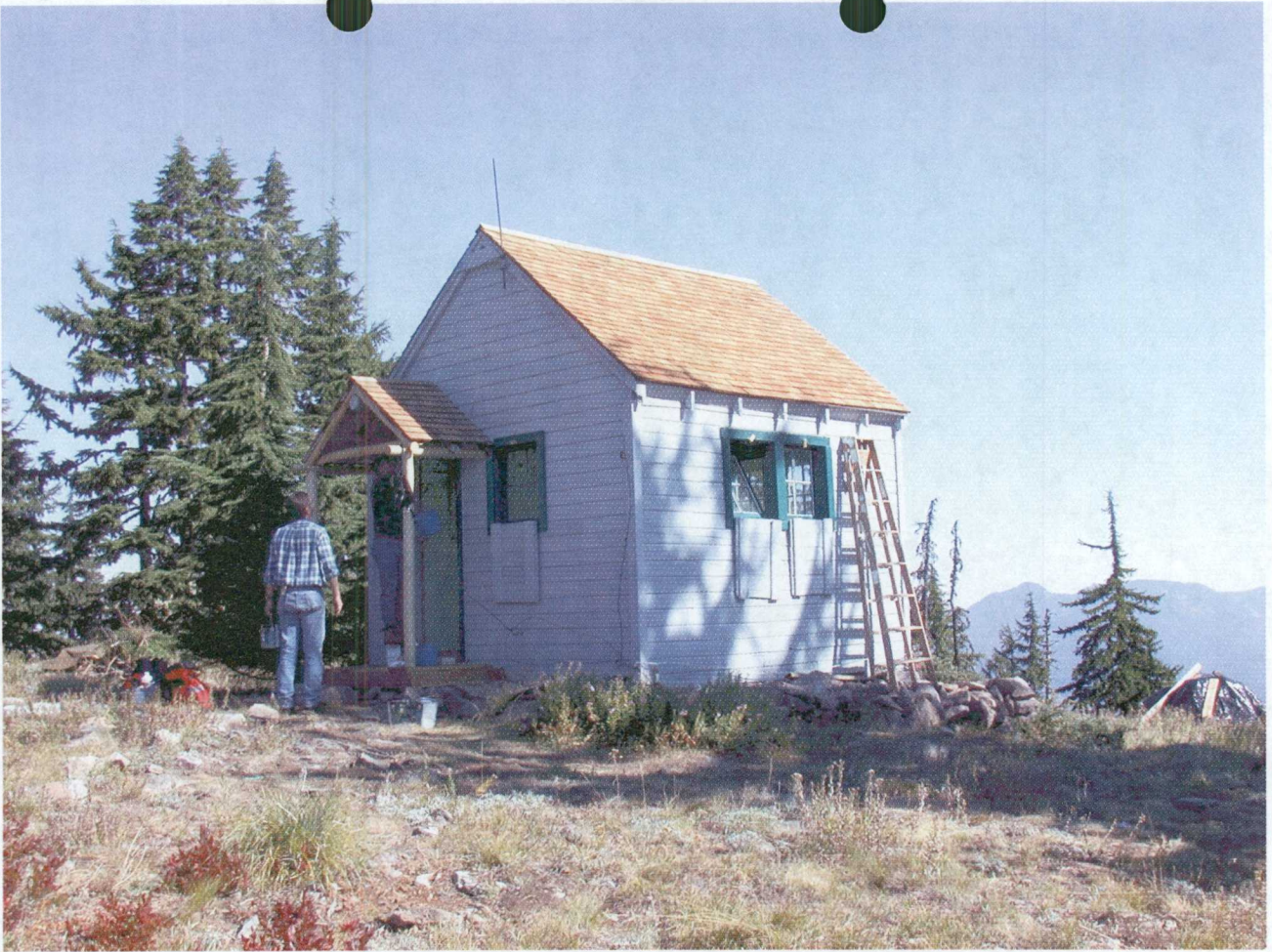
Cabin roof after completion
