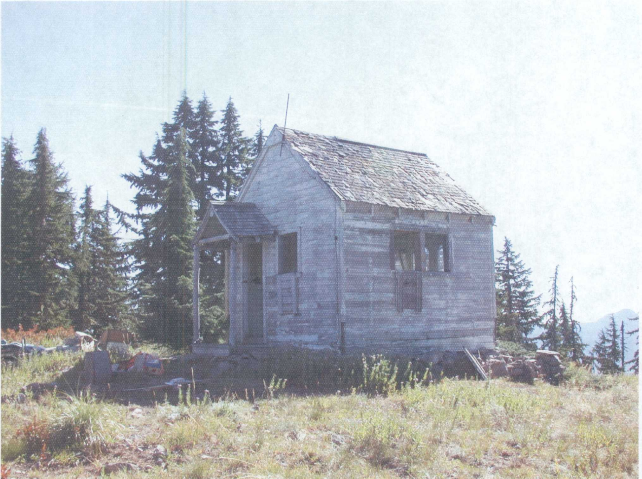
Cabin and roof prior to restoration
