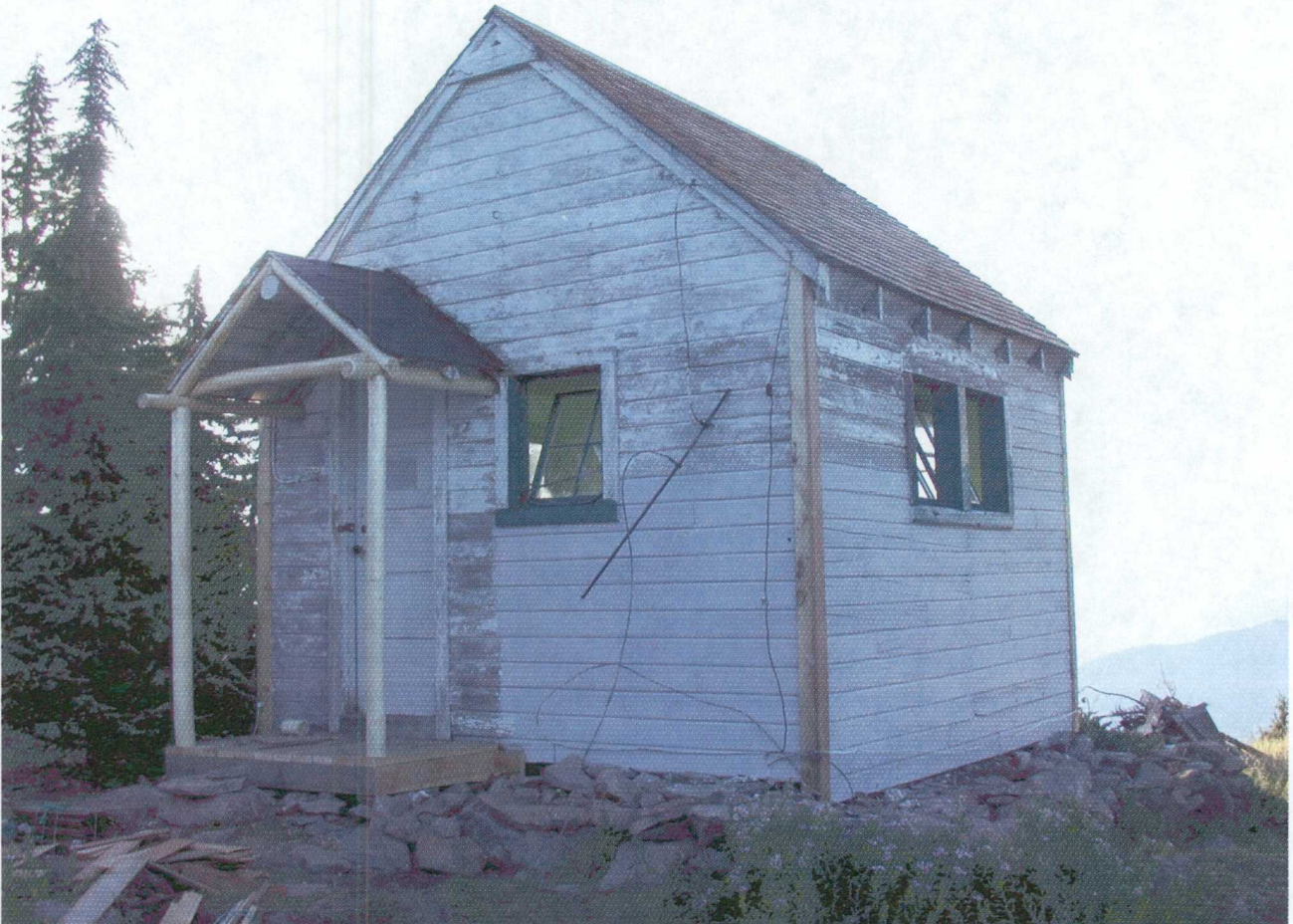
Corner trim and porch repairs
